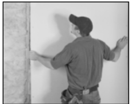
Figure 2.1: Install first layer of drywall
