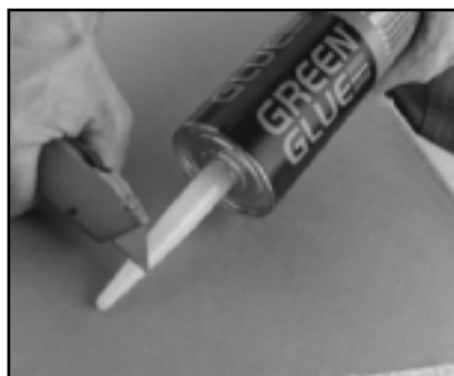
Figure 2.3: Cut a 3/8" opening in tube
