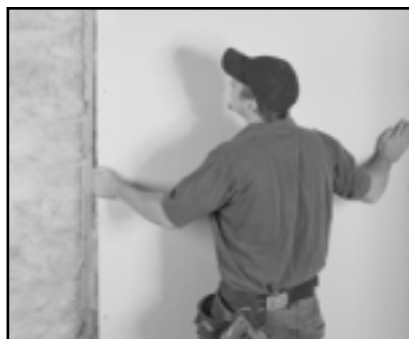
Figure 2.1: Install first layer of drywall
