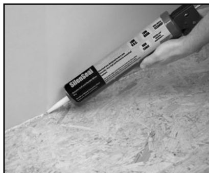
Figure 2.2: Use acoustical caulk along perimeter.
