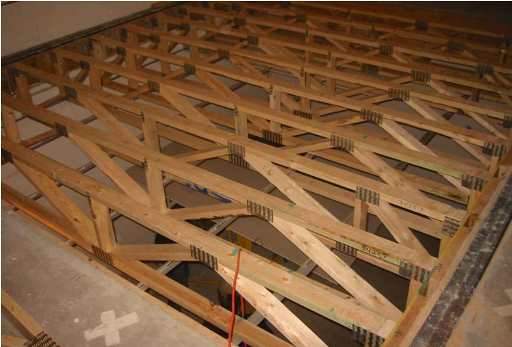
Figure 1: open-web truss joists
