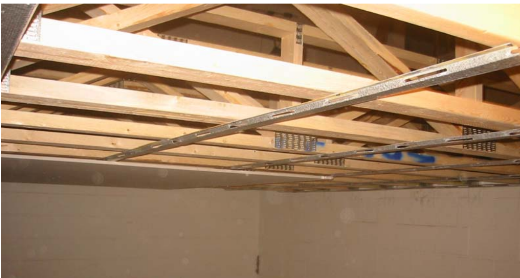
Figure 2: resilient channel and gypsum board ceiling
