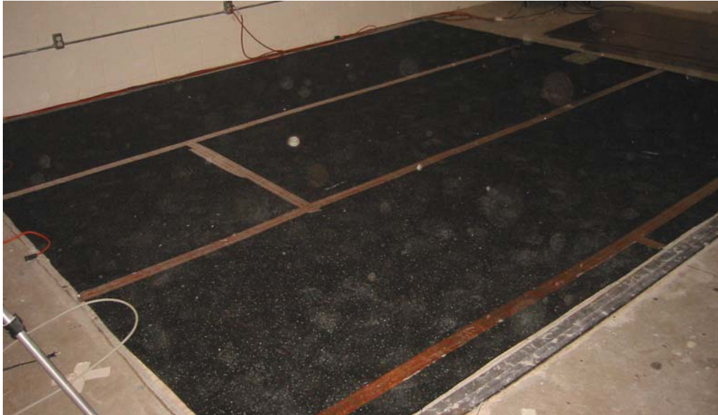
Figure 3: underlayment with foil tape
