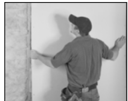
Install first layer of drywall
