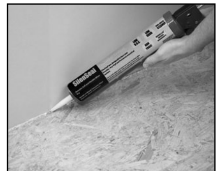
Use acoustical caulk along perimeter.
