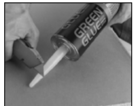
Cut a 3/8" or more opening in application nozzle.
